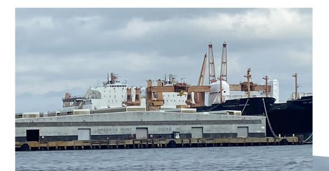
Lamberts Point Coal Terminal is an NS-served and operated transshipment terminal located on the Elizabeth River in Norfolk, Va. Annual throughput capacity is 48 million tons. The heart of the terminal is Pier 6, which has two shiploaders that permit the facility to load two vessels simultaneously. Twin tandem rotary dumpers feed the shiploaders for a combined dumping capacity of up to 8,000 tons per hour. Vessel loading rates are augmented by two surge silos.
