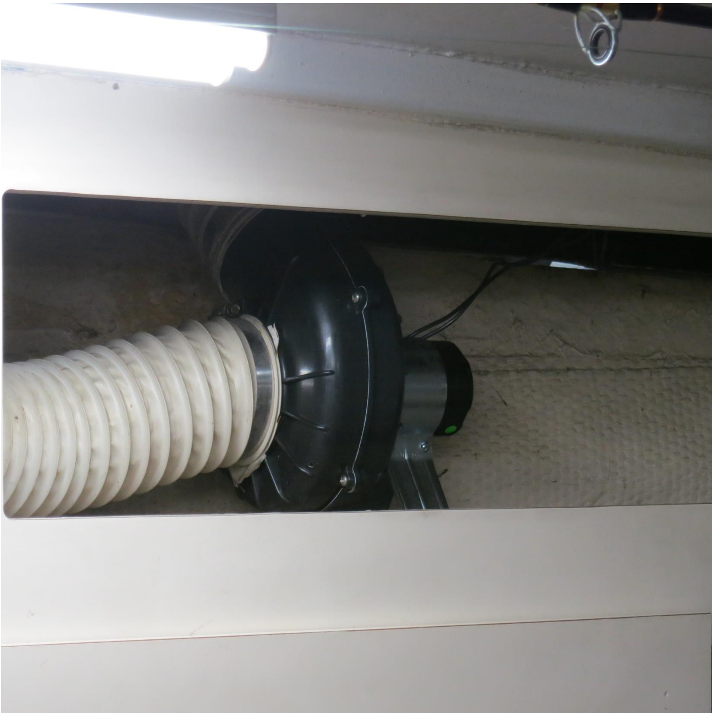
...A new exhaust fan.
