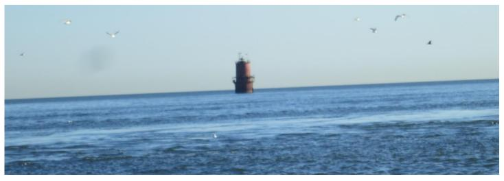
This lighthouse is the third lighthouse here on this spot and has been privately owned since 2004. It is a sparkplug lighthouse. A sparkplug lighthouse is a type of lighthouse that sits on a concrete or metal caisson. A caisson lighthouse which is also referred to as a sparkplug lighthouse usually has living quarters and is typically made of cast iron although not exclusively. A sparkplug lighthouse can also be known as a bug light.
