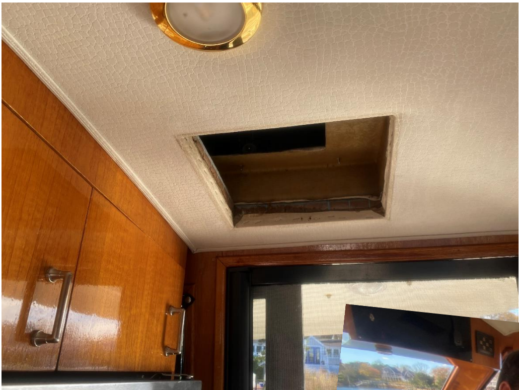
Valkyrie's galley vent.
