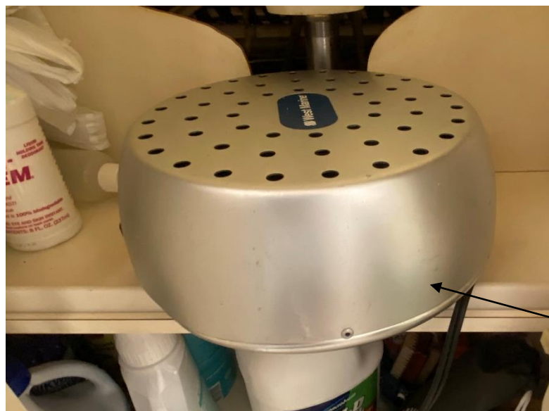
This is a small heater under the sink in Jordan's cabin. It is the lowest cabin on the boat so her pipes would freeze first.
